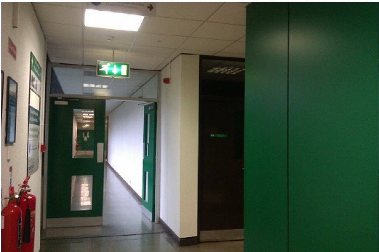
Room 220 is on the right as shown here opposite the fire extinguishers
